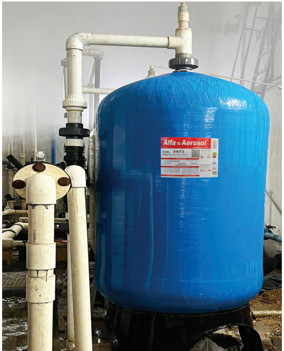
3672 FRP Pressure Vessel for Industrial RO Water Purification System installed in Le-Meridien
