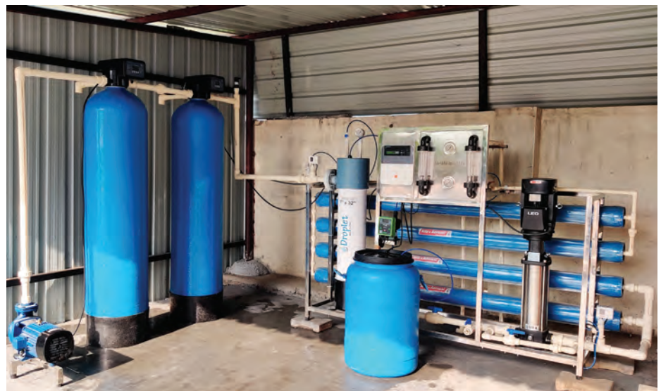
2000 LPH Fully Automatic RO Water Treatment Plant
