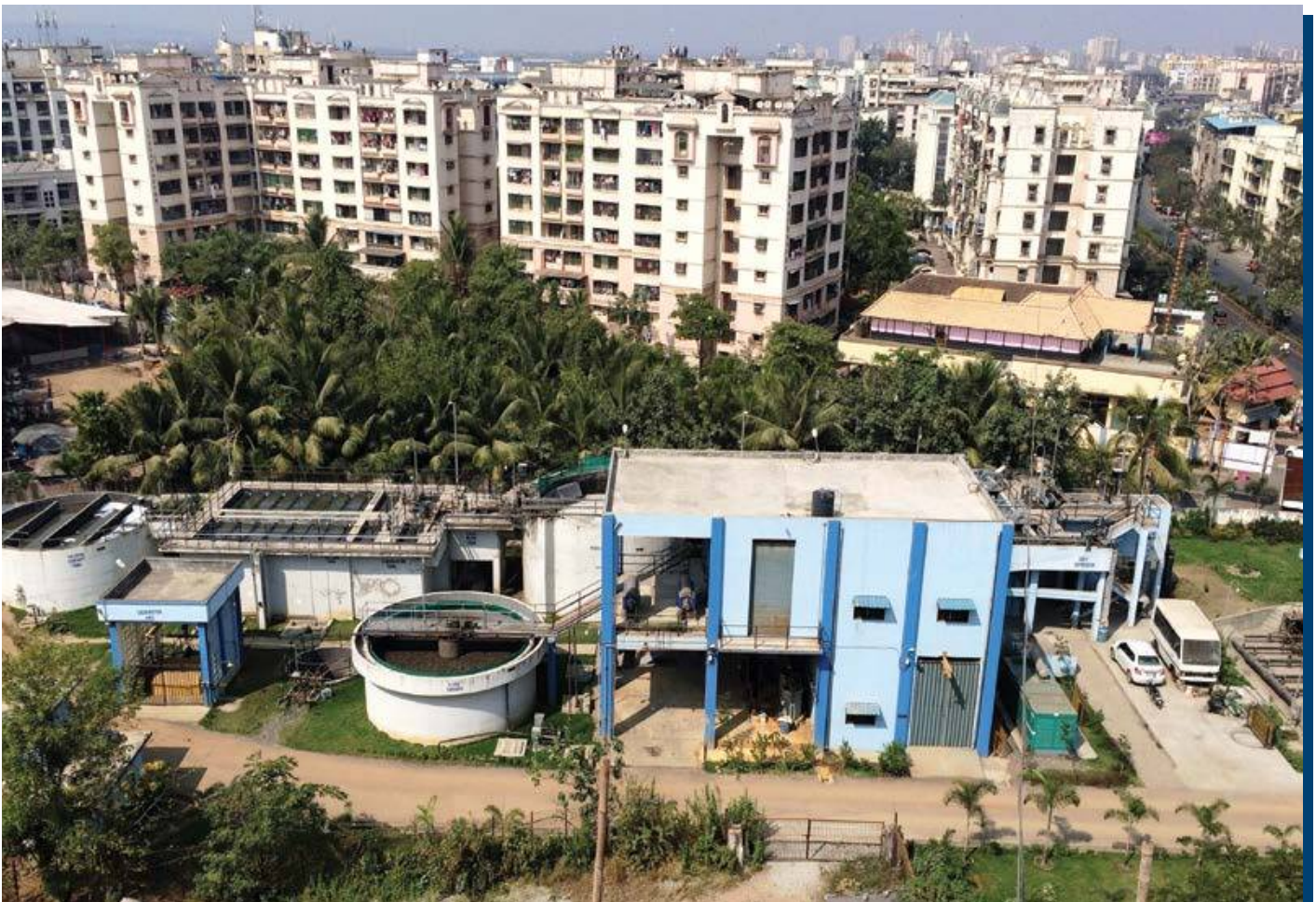
11 MLD Decentralised Sewage Treatment Plant, Mira Bhayander, Maharashtra
