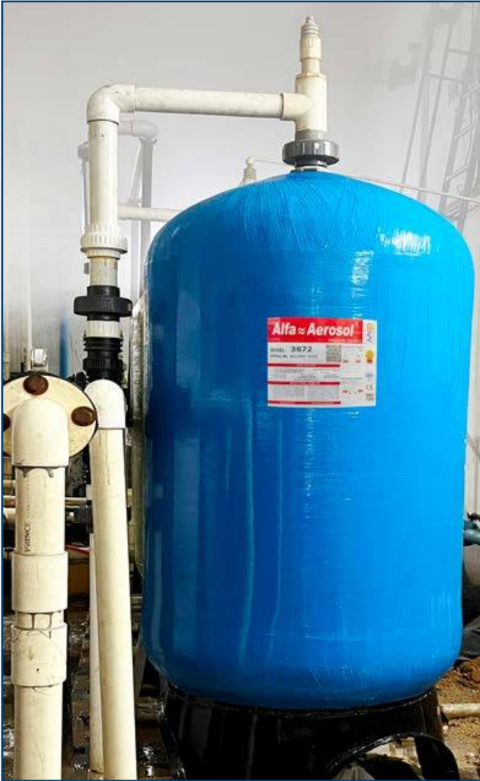
3672 FRP Pressure Vessel for Industrial RO Water Purification System installed in Le-Meridien
