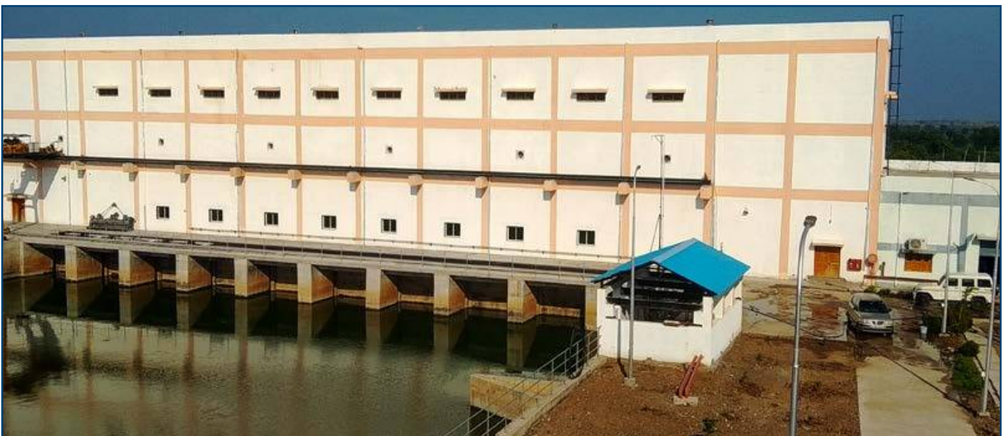
2587 MLD Pumping House for SAUNI Yojana Phase-1, Gujarat
