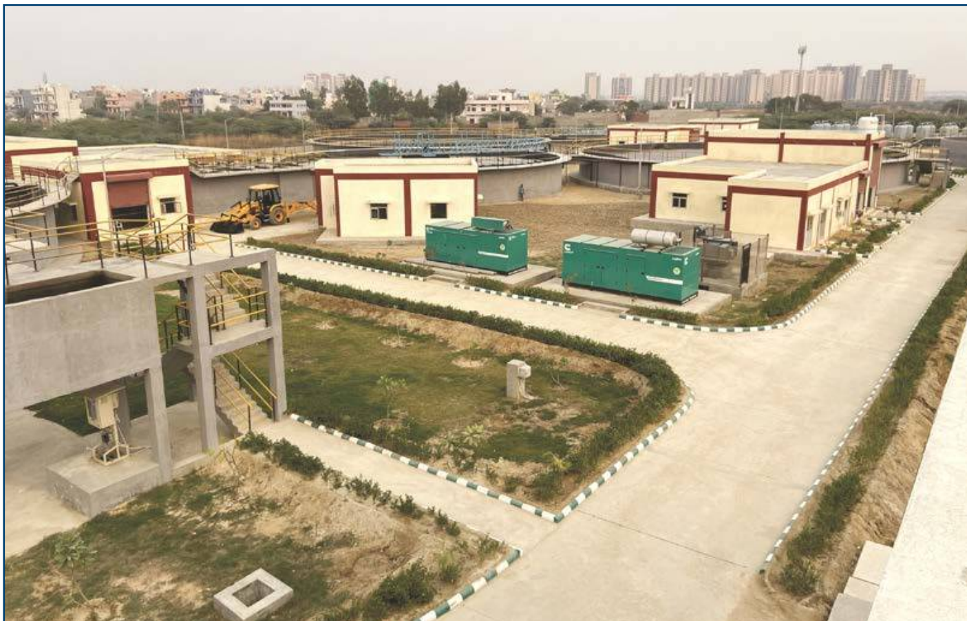
12.5 MLD Effluent Treatment Plant, Bahadurgarh Industrial Area, Haryana
