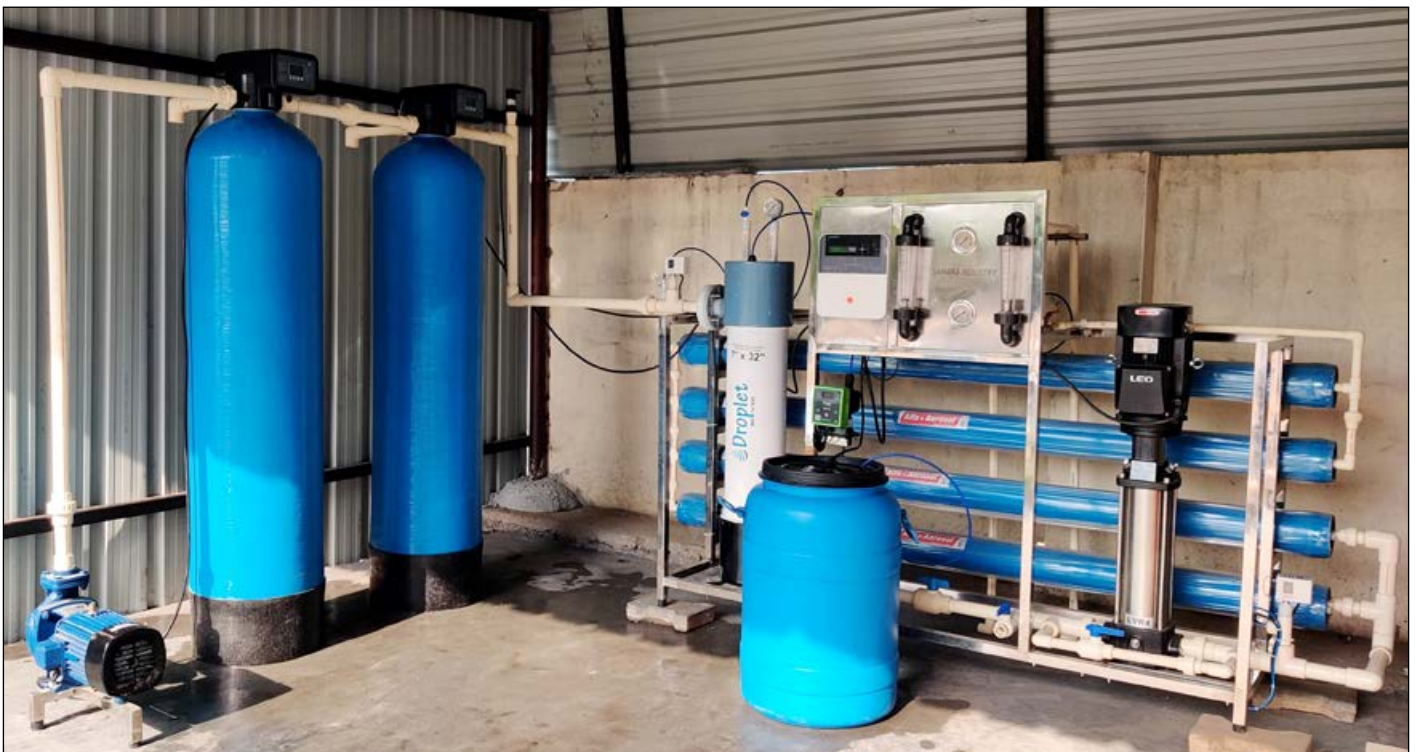
2000 LPH Fully Automatic RO Water Treatment Plant
