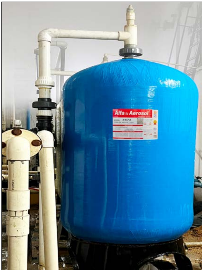
3672 FRP Pressure Vessel for Industrial RO Water Purification System installed in Le-Meridien
