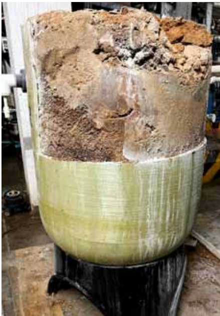
Pic 1.2-Cut Open Sand Filter Vessel at Le-Meridien
